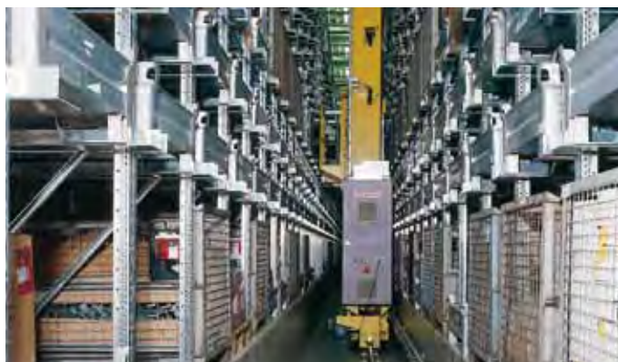
Automated pallet racking with single position storage
